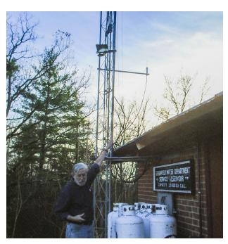
disconnecting the duplexer, using the existing antenna at the top of the tower for receiving only, and adding a temporary low-gain antenna inside the Water Department building for transmitting only. This solved the problem of the repeater transmitter desensing the receiver.
