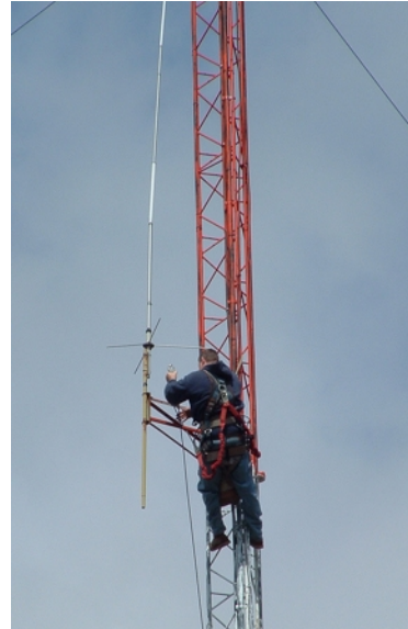
The tower climber replacing the coax cable
