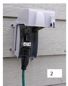
outdoor-rated extension cord goes to the generator, underneath the deck but in the open air where exhaust won't get into the house (Photo 3). The outlet box is rated for use in wet locations (Photo 4). Inside the house the special outlet is available for an extension cord to the pellet stove,
