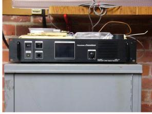
The new repeater contrasts physically with the old one. Backing up, you can see it in place. The old repeater, now unused, occupies with its power supplies most of the big gray cabinet the new repeater sits upon. The large light brown box to the left that looks like it could be a small refrigerator is actually a 2 meter duplexer. More on that below ...
